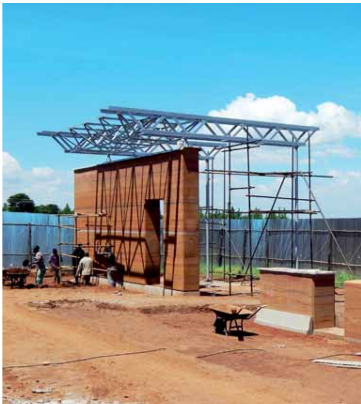
Fig. 16 – Vista del mock up della muratura in pisé. © Emergency NGO Technical Department
