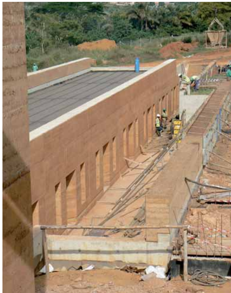
Fig. 22 – Costruzione delle murature in pisé. © Emergency NGO Technical Department
