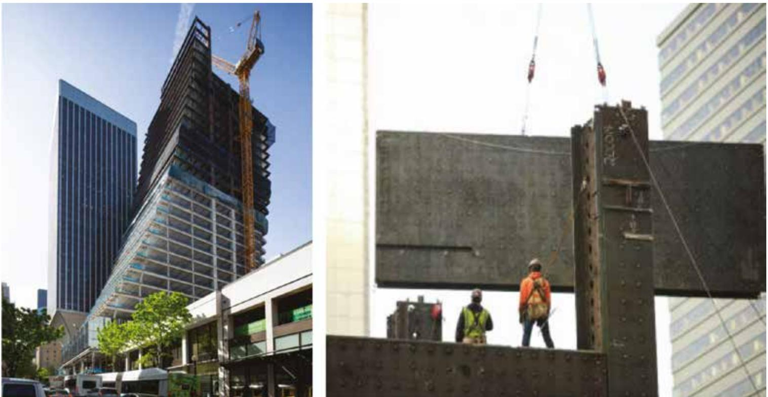
Fig. 9 | Construction of the composite core by crane lifting at Rainier Square Tower [32]
