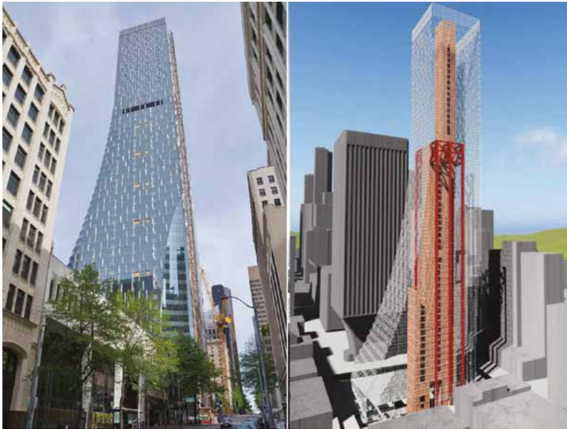
Fig. 8 | Rainier Square Tower, Seattle, USA (Mixed-use building, 260 m structural height / 58-floors / 1200 m<sup>2</sup> average gross area per floor), first major realization of the double-skin composite core SPEEDCORE [32]
