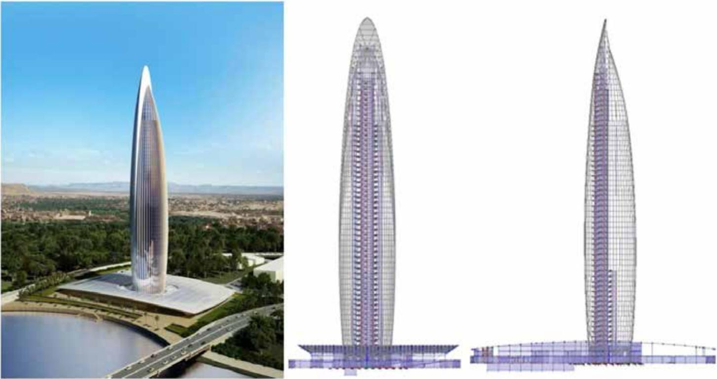
Fig. 15 | Rendering and view of the SCIA Engineer model of the Tour Mohammed VI in Rabat, Morocco – currently under construction (Mixed-use building, 250m structural height / 55-floors / 1300 m<sup>2</sup> typical gross area per floor).
