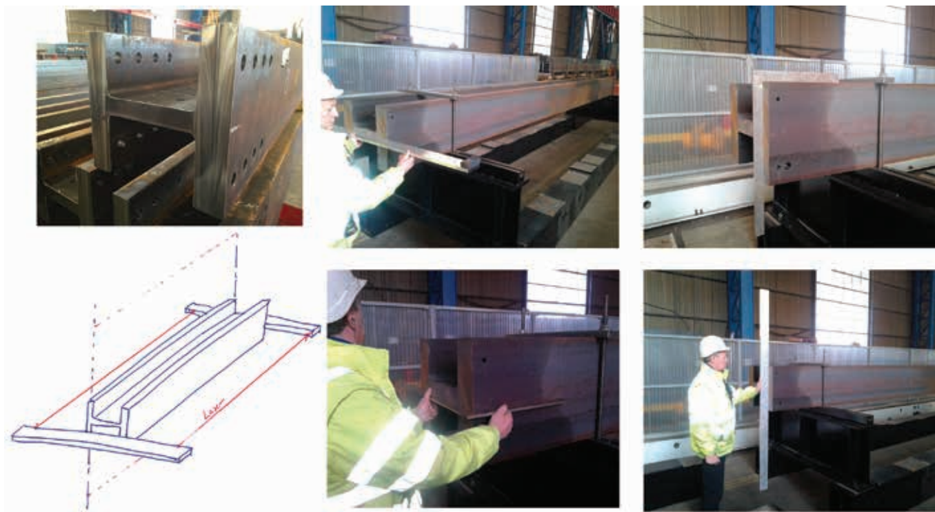
Fig. 8 | Example of quality control put in place after milling for a splice with direct contact
