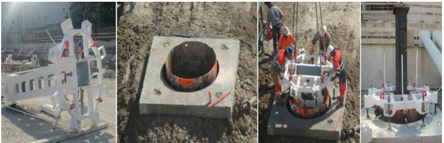
Fig. 13 | Example of guiding device fixed on the pipe head
