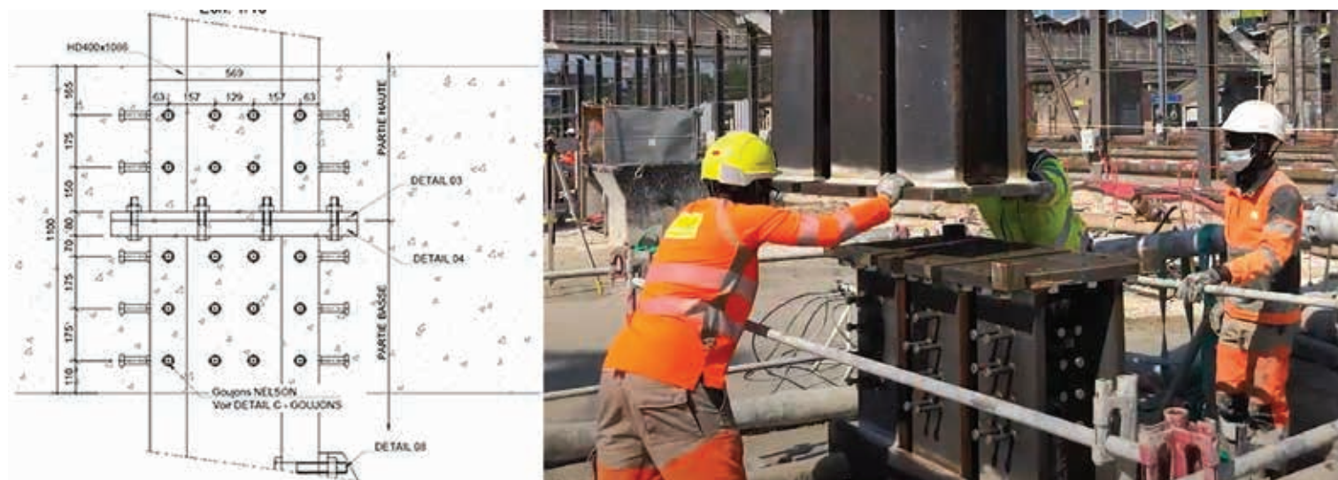
Fig. 9 | Splice by means of a headed plate foreseen at the slab level (left); erection on the construction site (right). Metro Line 18, Station of Massy-Palaiseau. Foundation at 43 m of depth, length of the plunge columns: 25 m. (Copyright: Spie Batignolle Fondations)
