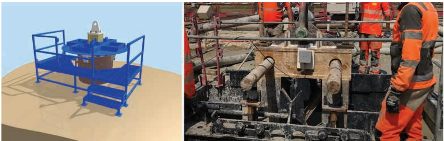
Fig. 15 | Blocking of the column top for the concrete phase
