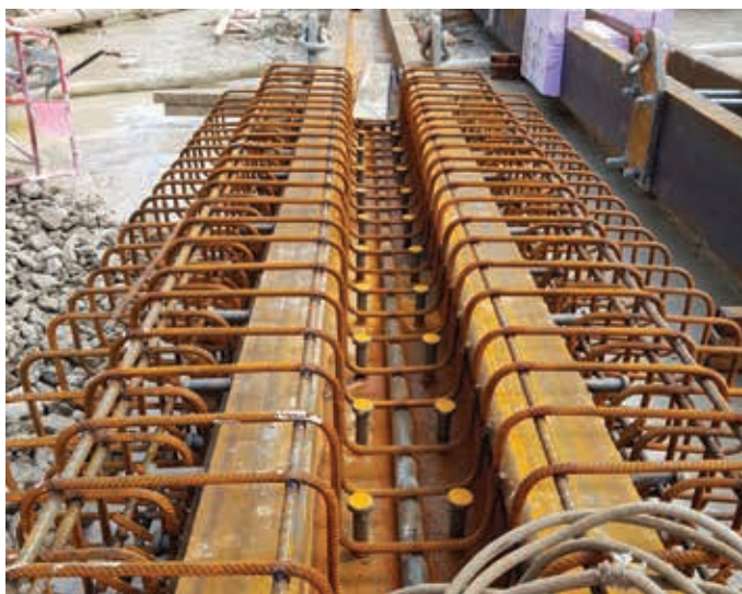
Fig. 11 | Shear connection by means of headed studs
