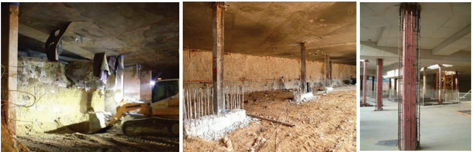
Fig. 3: View of the underground excavation (Left); Plunge columns after excavation (middle); steel column after removal of the temporary pipe and realization of the concrete slabs (Right) [7].
