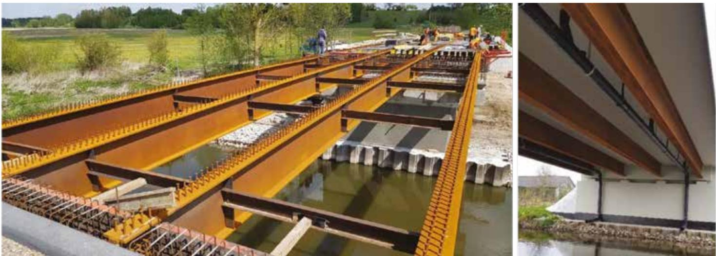
Fig.4 | (Left) Weathering steel girders at the erection of the composite bridge in Wirkowice (Poland) with a light orange-brown oxide layer after short exposure for several weeks; (right) after completion with an orange-brown oxide layer after exposure for six months
