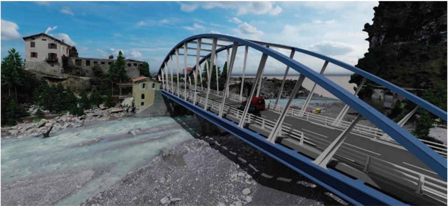
Fig. 6 | View of the central part of the decks with the hanger layout for the project considered
